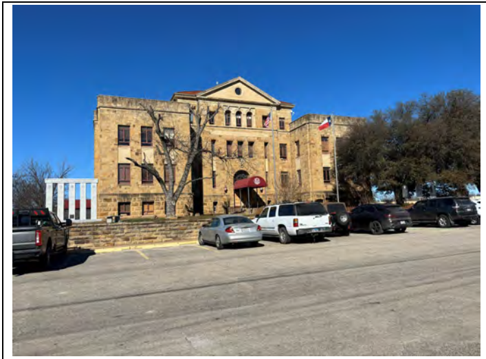
1. View of south side of Palo Pinto Courthouse
