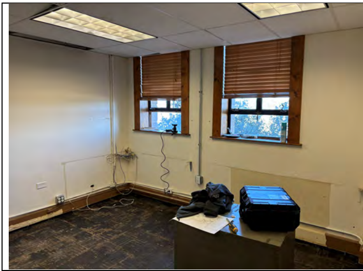
7. View of Room #4 on the 3 rd Floor.
