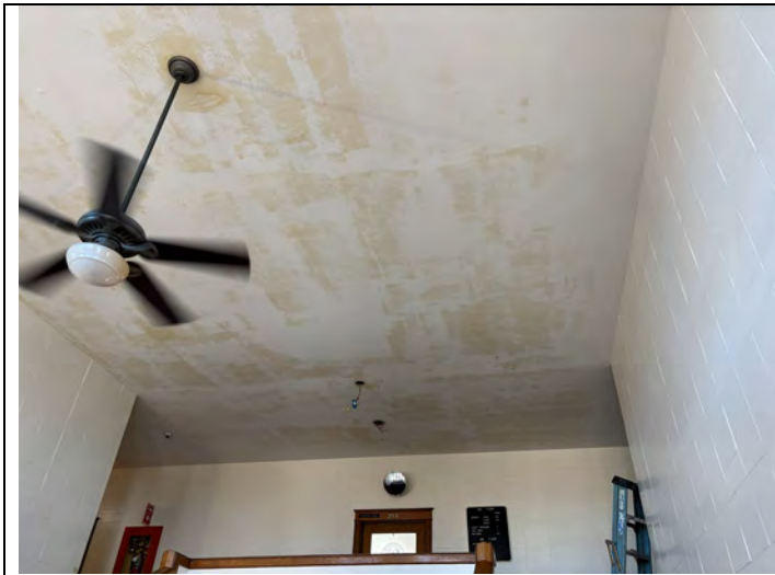
11. View of hallway ceiling above stairwell on the 2 nd Floor.
