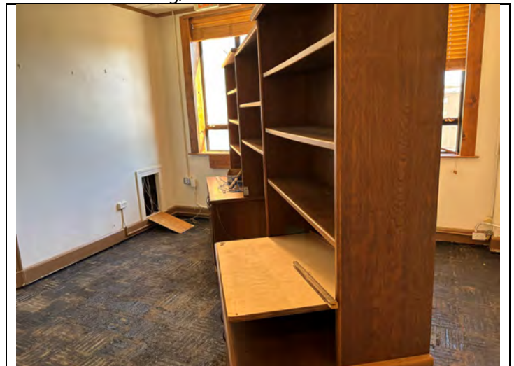
6. Room #2 on the 3 rd Floor
